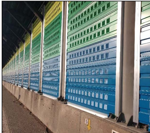
⑤ COVER PLATE INSTALL
