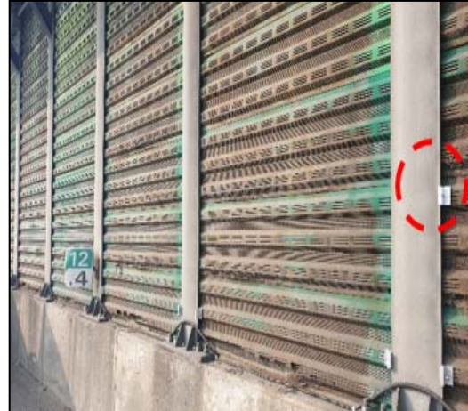
② FIXING ANGLE INSTALL
