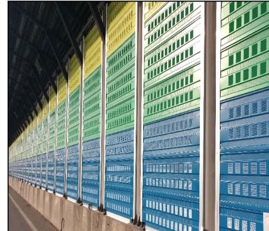
⑥ AFTER REMODELING
